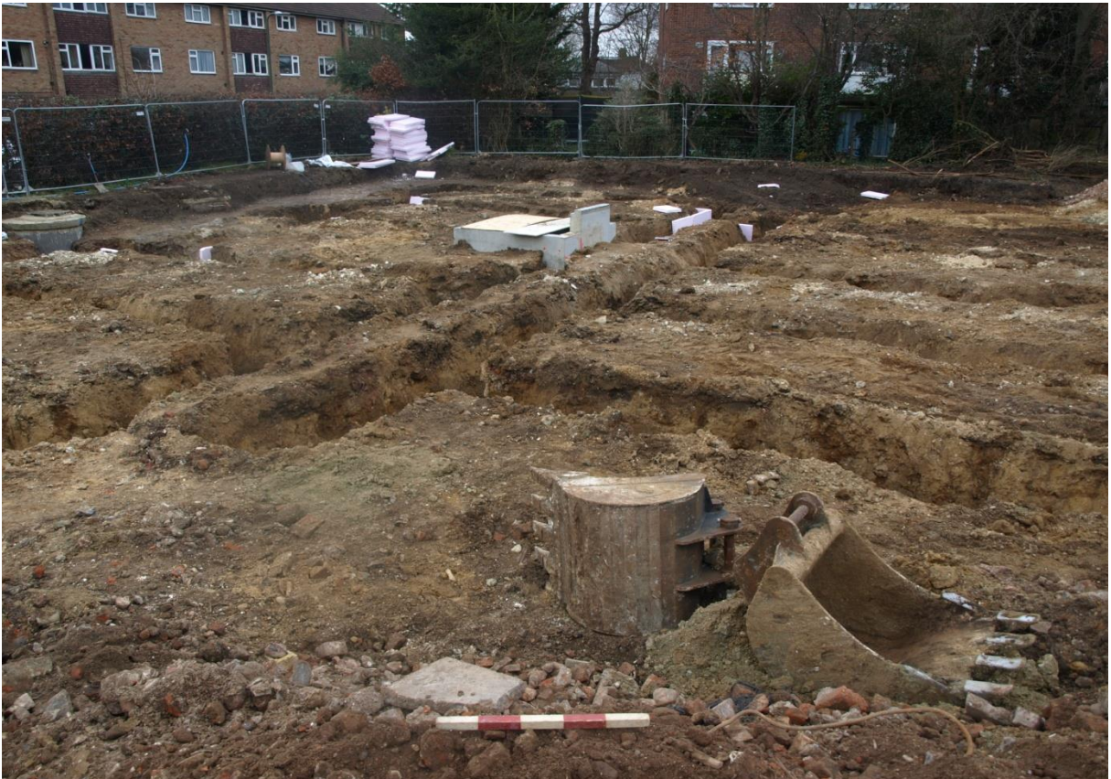
Plate 17: Showing foundation trenches, viewed from the northeast
